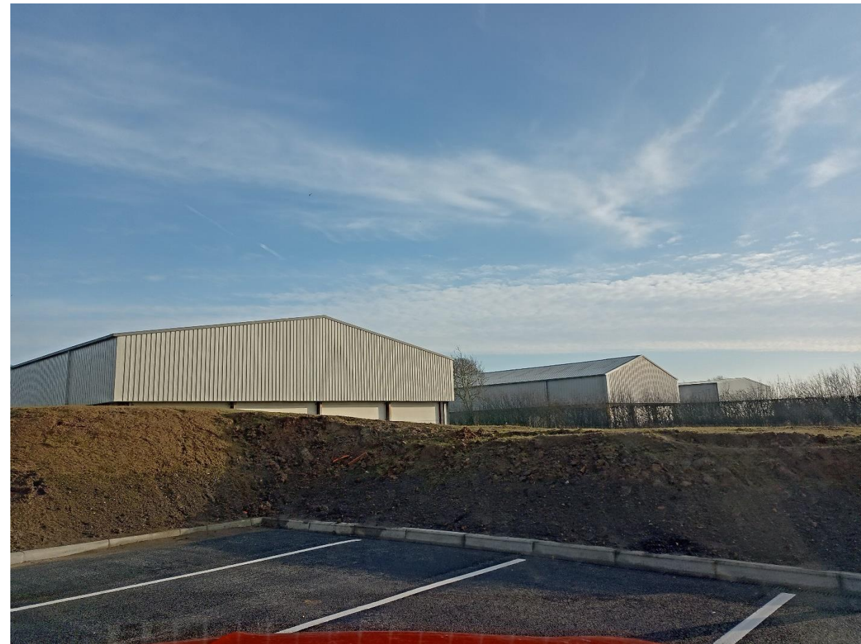
Rear elevation of Buildings
