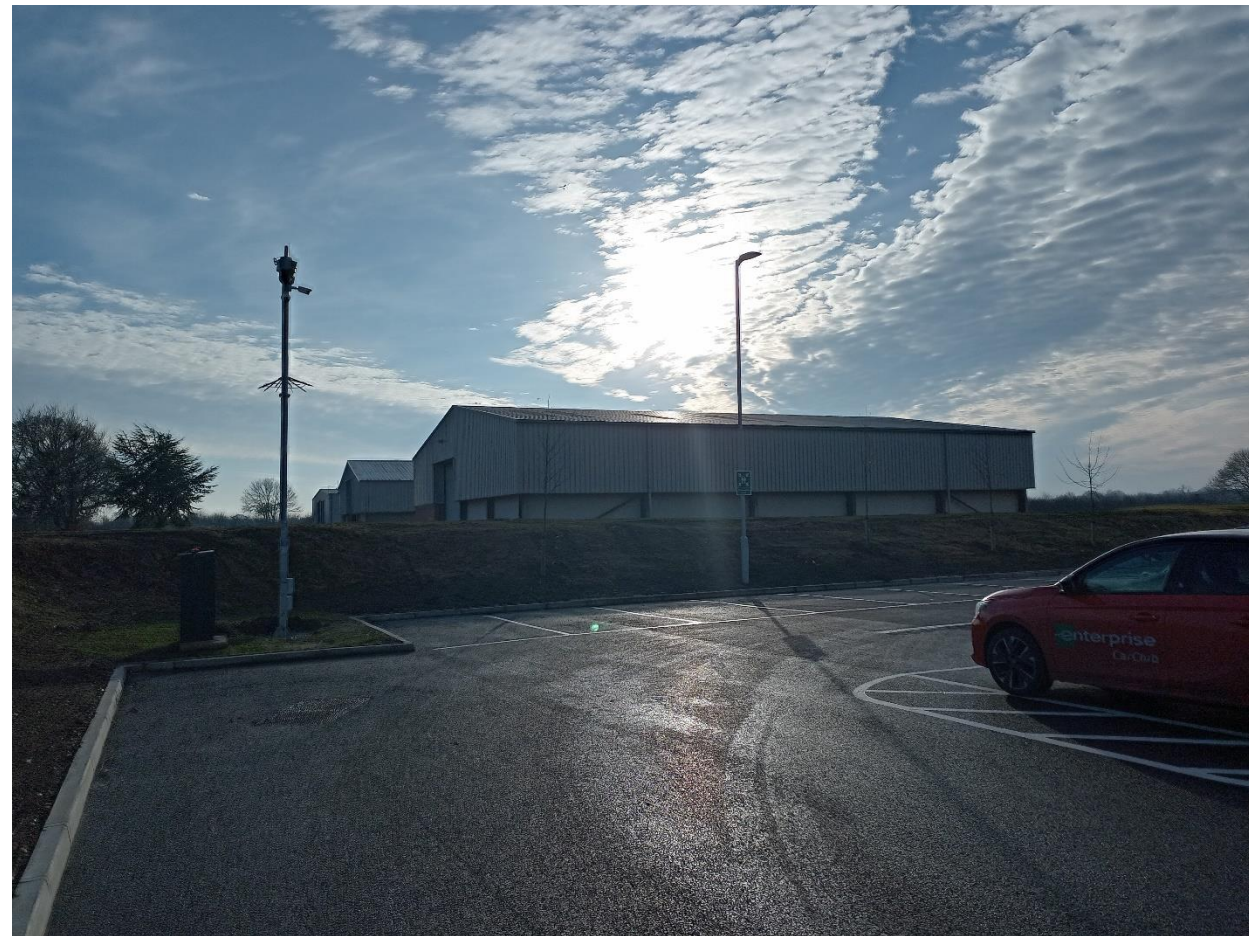
View from neighbouring DPD Car Park
